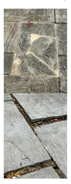
2.4 Image 4 above (bottom right-hand quartile) shows the extent to which the slabs have moved near the vehicle gated entrance immediately alongside Cockpit Path car park.
